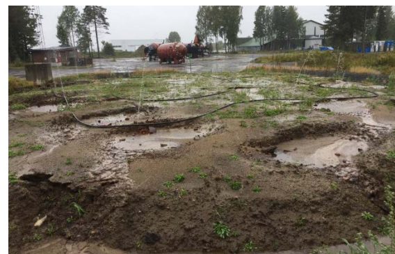
Test project with the washing of PFOS-contaminated soil
