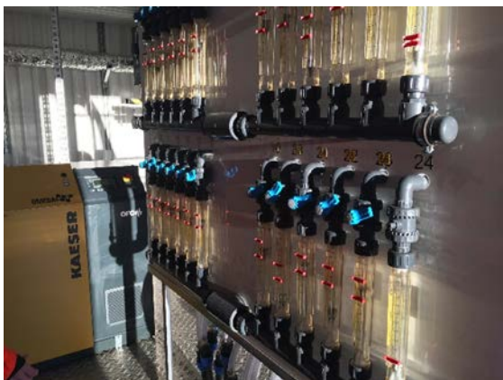
Management of air injection
