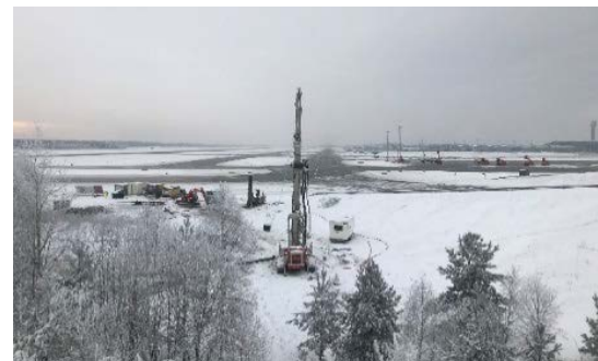
Drilling for thermal rock energy
