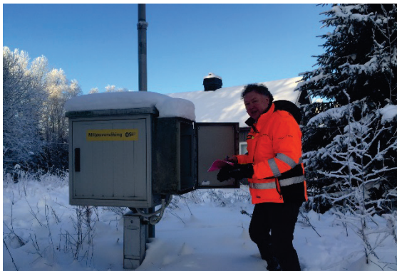
OSL's NTMS records the aircraft noise level continuously at 11 points around the airport
