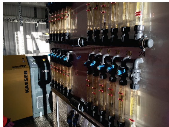
Management of air injection
