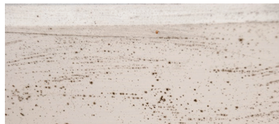
Blackening of buildings is due to mould growth, not emissions from aircraft
