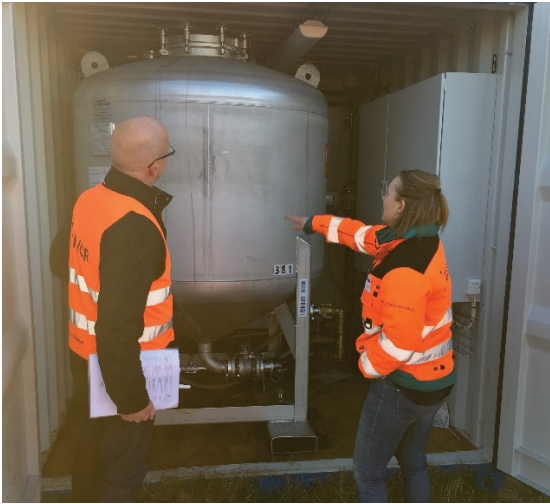
The PFOS treatment plant, container solution
