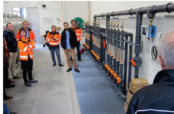
The groundwater treatment plant for PFOS at the OSL fire drill facility
