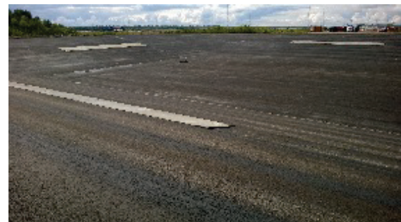
The snow storage facility is ready to receive the winter's snow
