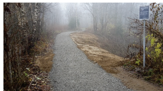
Clearing up the unofficial dumping ground in the Romerike nature conservation area
