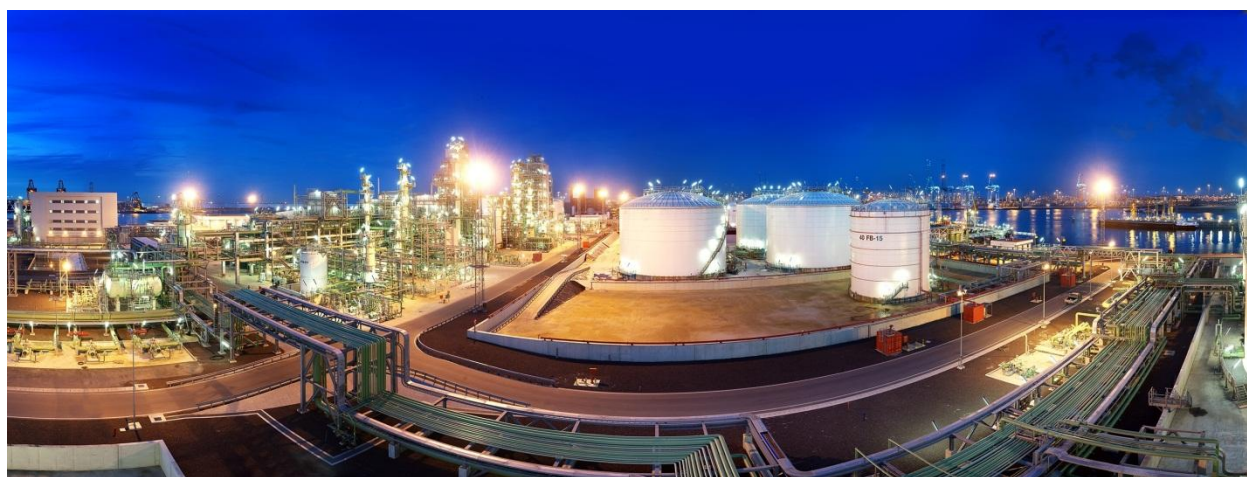
Figure III – Bio refinery and storage tanks © Neste Oil
